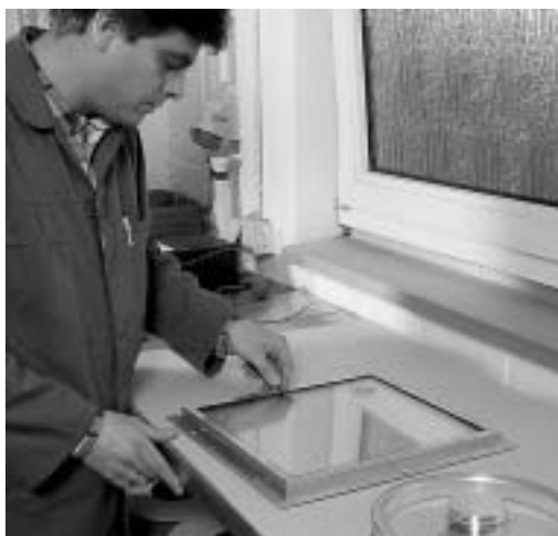
Thorough cleaning of the polycarbonate pane
